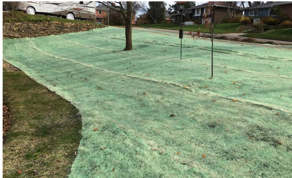
*Erosion mats installed on slope after native seed was installed underneath. Young plants will grow through the mats.*
